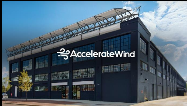
The building accelerate the wind
