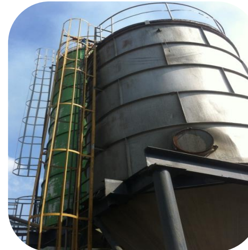
Vegetable oil waste treatment Q=80 cubic meters per 5 days
